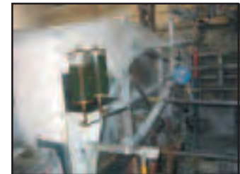
Gravity feed oilers on a mud washing drum
