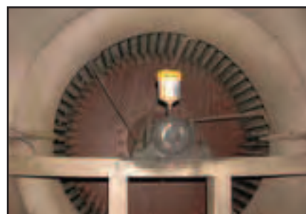
Streamliner V installed on a blower fan
