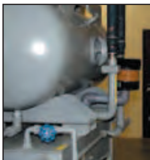
Watchdog Breather installed on a hydraulic reservoir
