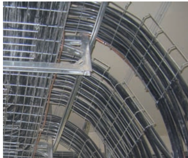
INSIDE/OUTSIDE BENDS - CHANGE OF PLAN adjustable on site
