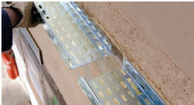
Fit the cable tray...
