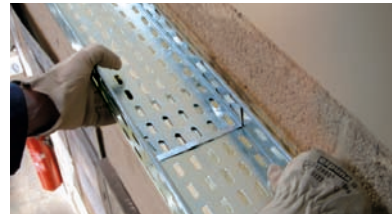
Pull up to locking position
