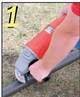
1 Clean pipe before making weld.
