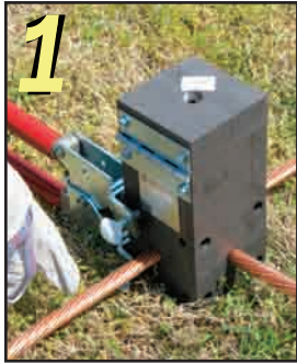
Position cleaned conductors in mold
