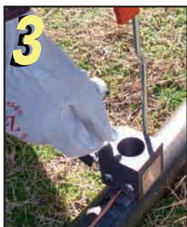
3 Place metal disc in bottom of mold.
