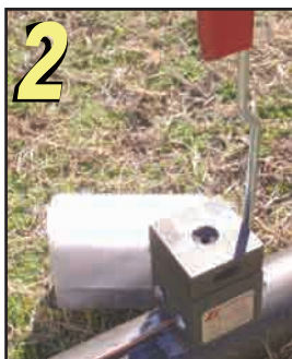
2 Position conductor and mold onto pipe.
