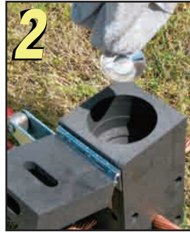
Place metal disc in bottom of mold crucible.
