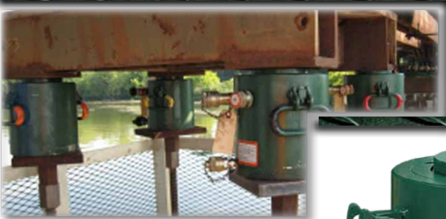
These 100 ton RCD cylinders are being used to construct grid sections for a bridge being built over the Susquehanna River at the mouth of the Chesapeake Bay.
