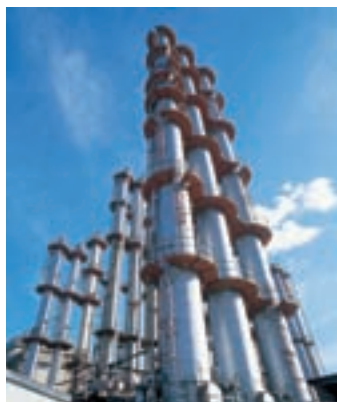
High temperature heating medium
