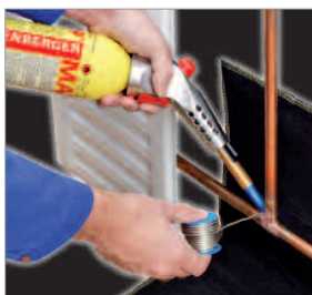
Soft soldering in heating installation
