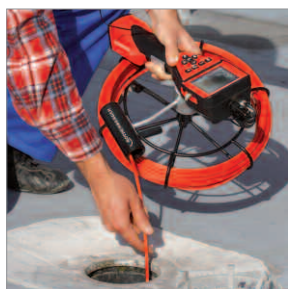
Inspection of rain downpipes
