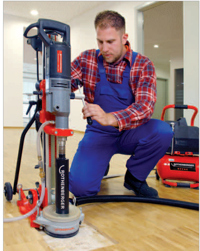
Clean work in enclosed rooms
