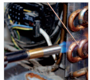
Hard soldering in refrigeration and climate control
