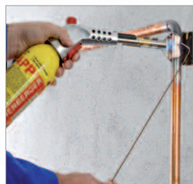
Brazing in gas installation
