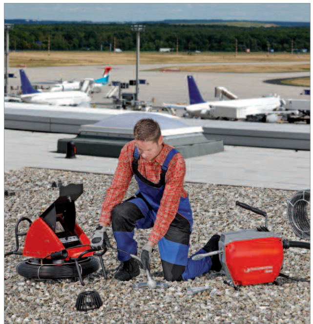
Inspection of a rainfall drains
