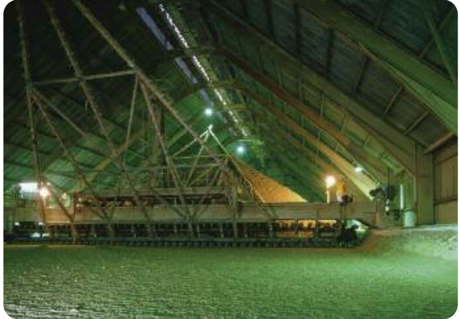
Clay/Limestone Store showing stacker and reclaimer. Max. capacity 43000 tonnes, rail dia. 88m.
