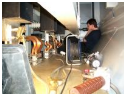
Installing couplers on site
