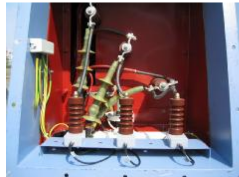
Couplers CC14B installed on a motor terminal box
