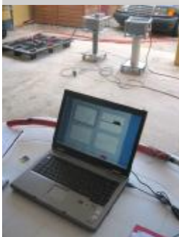
On-site cable testing
