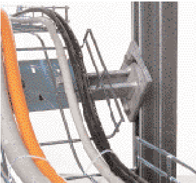
Fixing of Cable Trays
