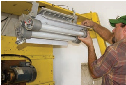
4. Replace with a new globe assembly in the reverse order. Feed the wires back into the globe ends & bolt in place.
