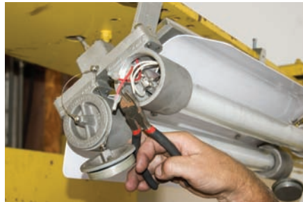
2. Remove the end caps and cut the wire connections.
