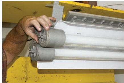
5. Rewire as per the diagram provided with the replacement globe. Check for proper lamp installation and replace end caps.
