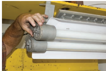
5. Rewire as per the diagram provided with the replacement globe. Check for proper lamp installation and replace end caps.
