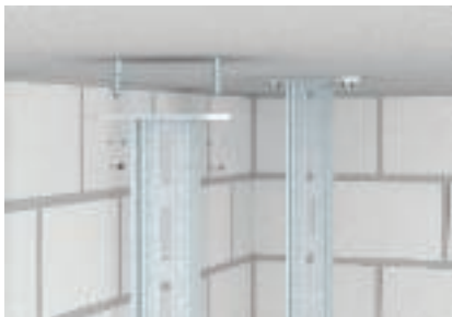
Installation of I support Standard mounting of I supports using anchor bolt, type FAZ II, to concrete ceiling.
