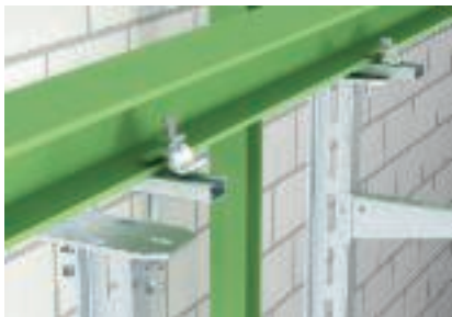
Steel clamping with C profile, tray in longitudinal direction I support with welded head plate mounting, clamped to steel girder with C profile and TKH-L-25 chuck jaw. Tray route along steel girder.
