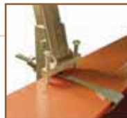
Stanchion installation complete
