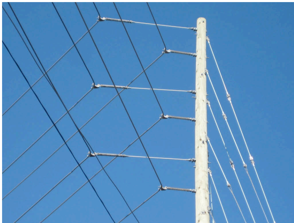
Extension Link Insulators in Vertical Corner Installation
