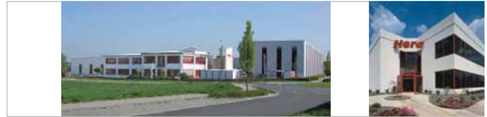
Hera headquarters in Enger, Germany
