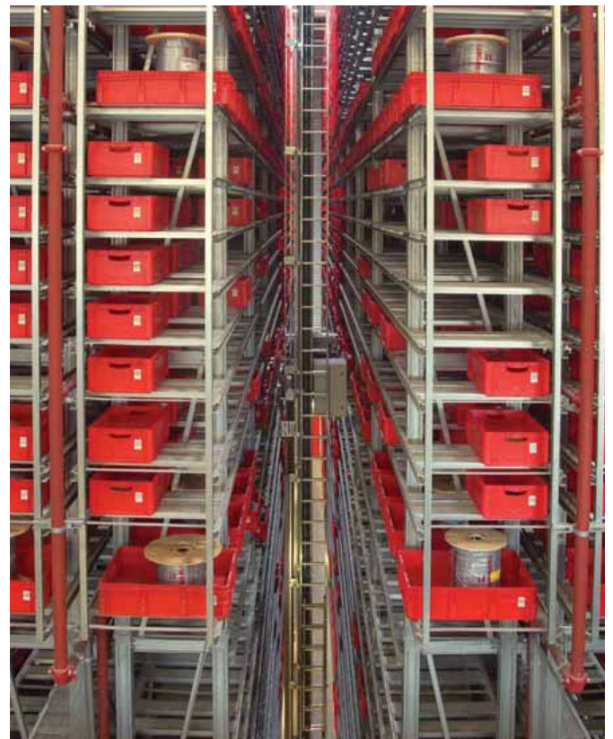
Small parts warehouse
