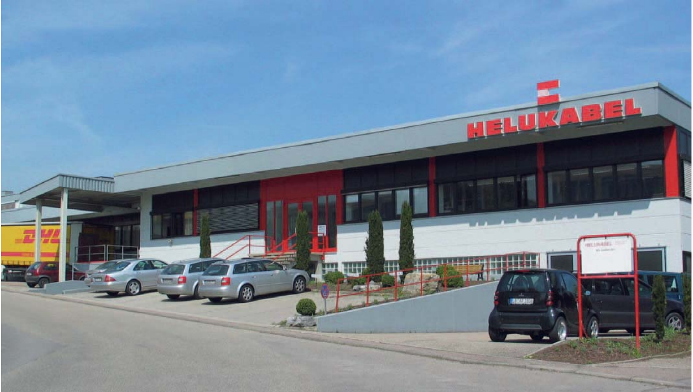
Photo: HELUKABEL® – Headquarters Hemmingen
