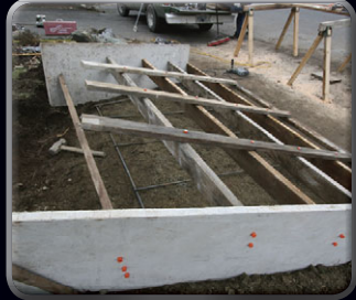
Stronger forms, less bracing
