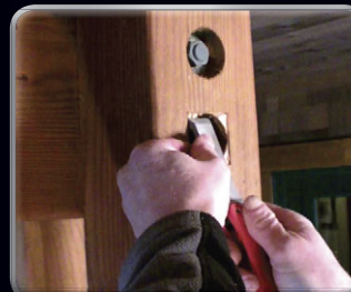
A Pocket Chisel creates square corners for the accent
