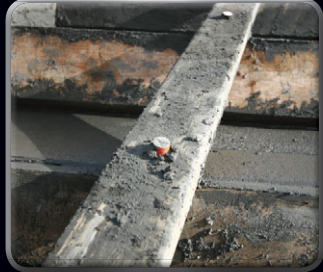
Great for vertical bracing
