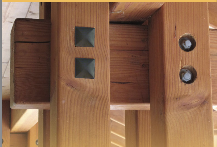
The 2" Artisan Chisel on an air hammer leaves a perfect outline for the Accents.
