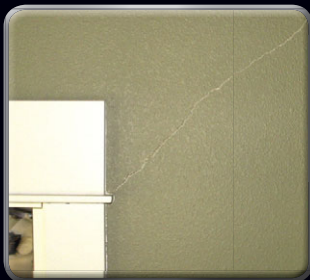
Stress Crack
