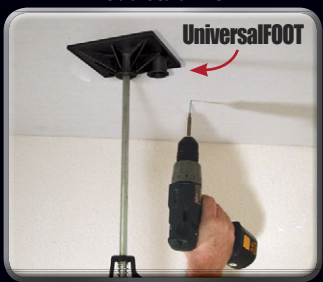
Drywall install with UniversalFOOT
