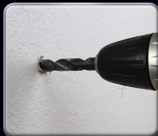
Use a 1/2" drill bit to bore a hole
