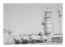
The design is suitable for both vacuum and gas stripping applications with corrosion resistant tower internals designed for foam retention, efficient liquid and gas phase distribution and redistribution, in order to maximize mass transfer efficiency.
