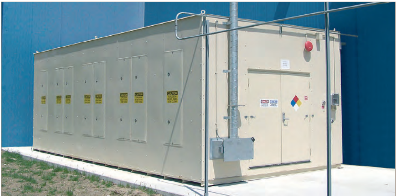
Heated and cooled Storage Building with fire suppression system, fire rated construction, and explosion-relief panels designed to house automotive paint pumping equipment
