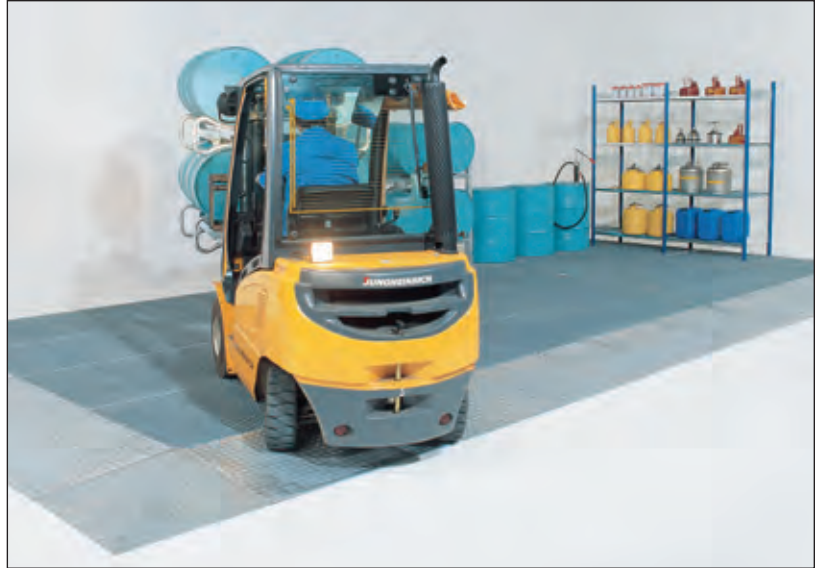
Custom constructed Spill Decks allow for truck and forklift access
