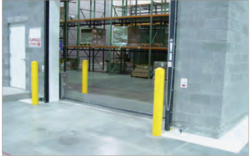
Automatic Doorway Spill Barriers are often utilized as containment equipment for Flammables Storage Rooms
