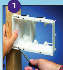
1 Attach box to stud. Use tabs for proper positioning of box depth. See Photo A .
