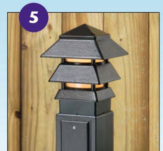
6 Install pagoda light to post with locknut inside the top of the post. Wire fixture.
