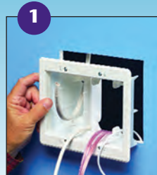
1 Using box as a template (without trim plate), mark location. Cut drywall. Attach trim plate to box. See Photo B . Install box assembly in opening.
