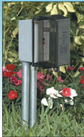
Why Install Boxes This Way...
