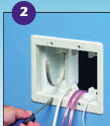
2 Tighten mounting wing screws to pull the box securely against the wall board. See Photo B .
