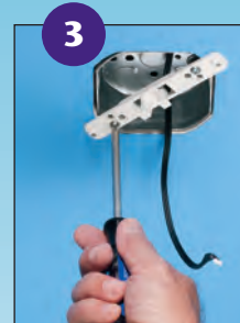
3 Mount the bracket to the existing box using screws provided.
